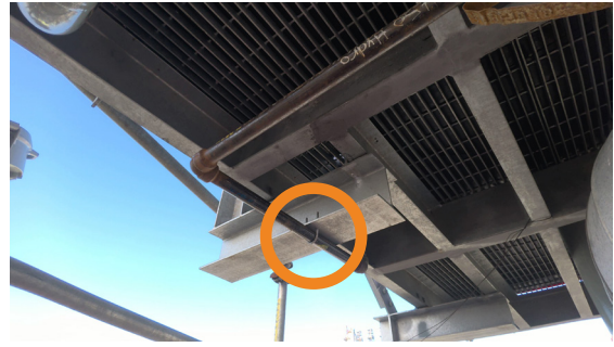
Fig. 3 Installed U-Bolt
