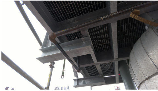
Fig. 2 Missing U-Bolt
