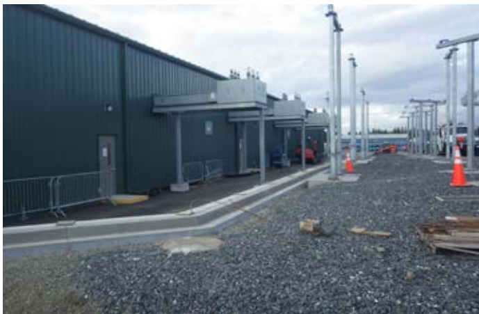
Figure 7. Completed Pre-Engineered Metal Building
