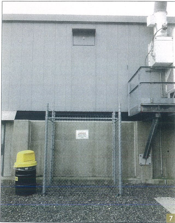
An isolation zone for blast vents. (Used with permission from BP.)
